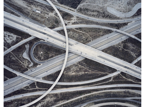
Highway overpasses in Atlanta, Georgia.
